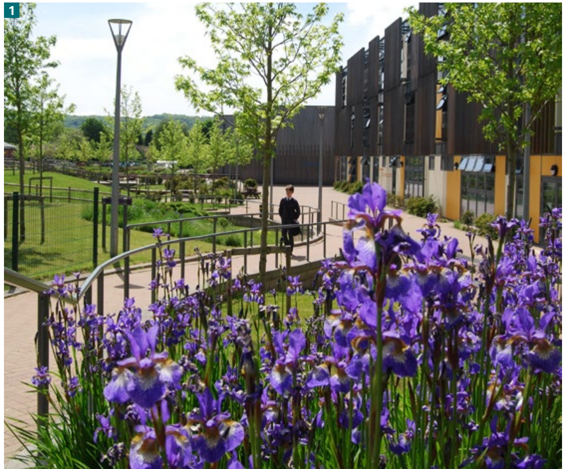
1. Rednock School, Illman Young Landscape Design Limited, 2010. Planted swale integrated within the open space design for a school.
