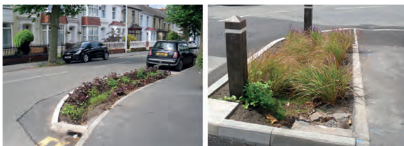
Figure 10. Examples of bioretention systems providing traffic calming measures, Llanelli, Dŵr Cymru Welsh Water 46 Using SuDS to improve the streetscape, providing multi-functionality by integrating with other street features including tree planting, traffic calming, parking bays, verges and central reservations.
