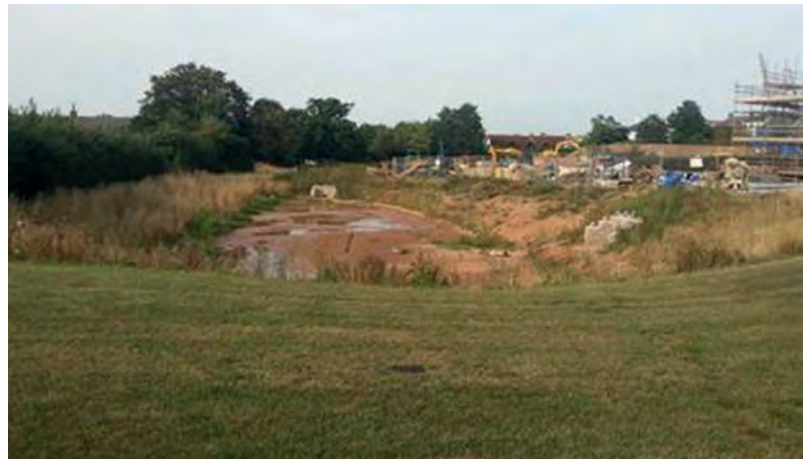
Figure 3. Somerset, a missed opportunity for SuDS. Photo courtesy of Peter Melville Shreeve. The 'lake' on this housing estate of 200 homes is always empty and unsightly. The lake will only fill during a one in 100-year storm event. This could easily have been designed with higher amenity value, as useable space, but the plans already had decided on the pond before drainage consultants were engaged on the design.
