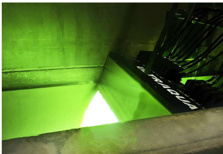
Figure 2 – Ultraviolet (UV) radiation facility being used for treatment.
