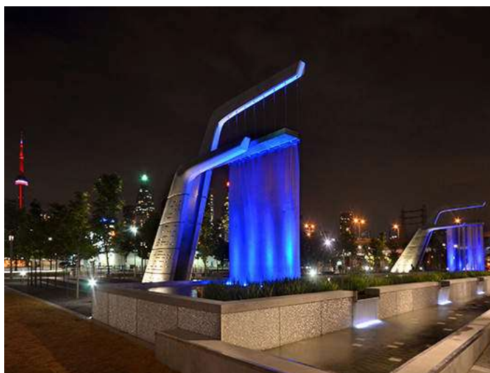
Figure 7 – UV Stormwater treatment facility, Ontario
