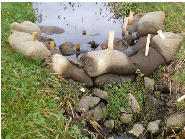
Figure 8 – Mycofiltration for urban stormwater treatment
