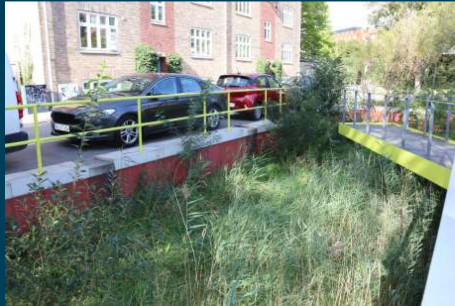
Surface system - treated in biofiltration systems
