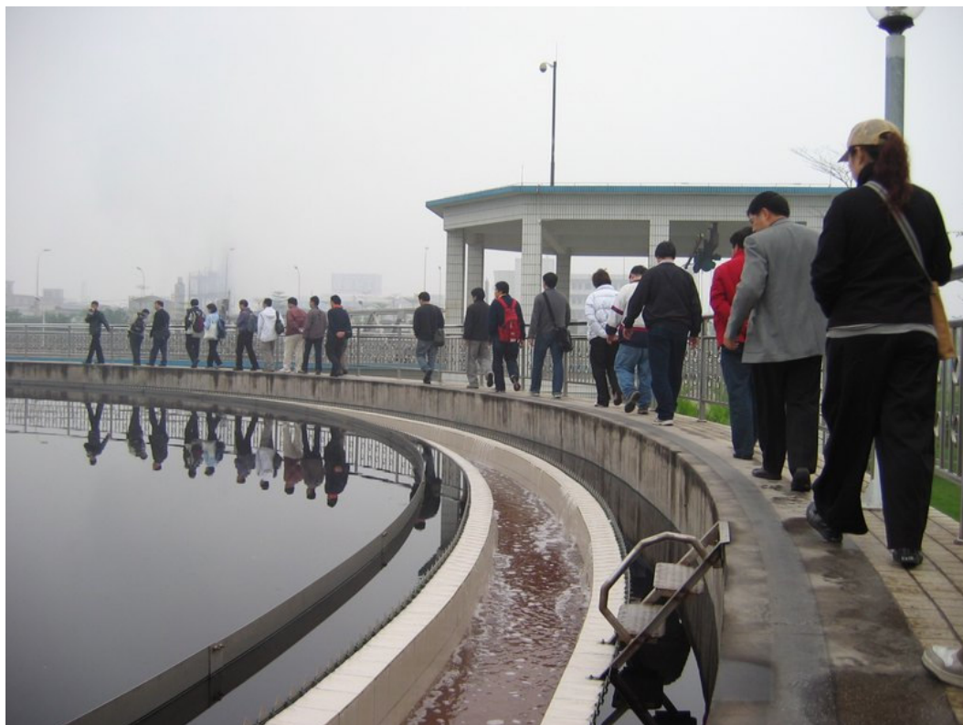
Visit to the First Municipal Sewage Treatment Work
