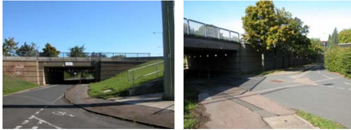
Gunnels Wood 'sunken' roundabout – Pocket Park - before
