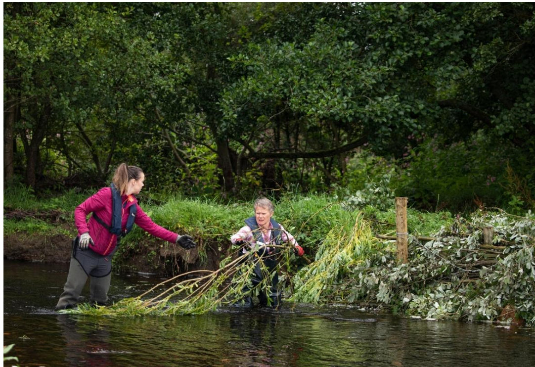
Volunteers spiling willow to stabilise river banks
