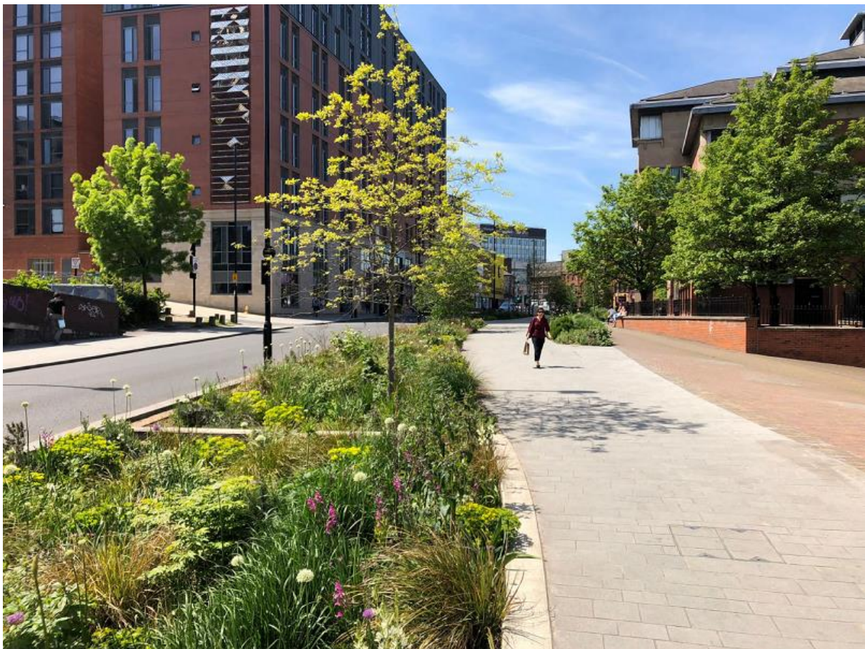
SuDS in the Sheffield Grey to Green retrofit scheme (photo: George Warren)
