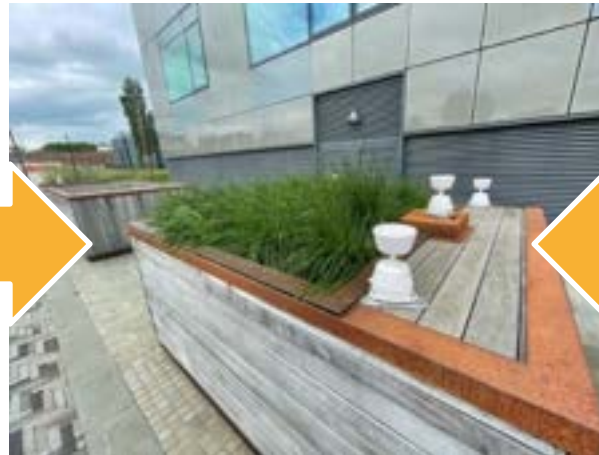
Bioretention Lysimeters (NGIF) Collection of: ◆ Long-term validation data ◆ Controlled design storm simulations
